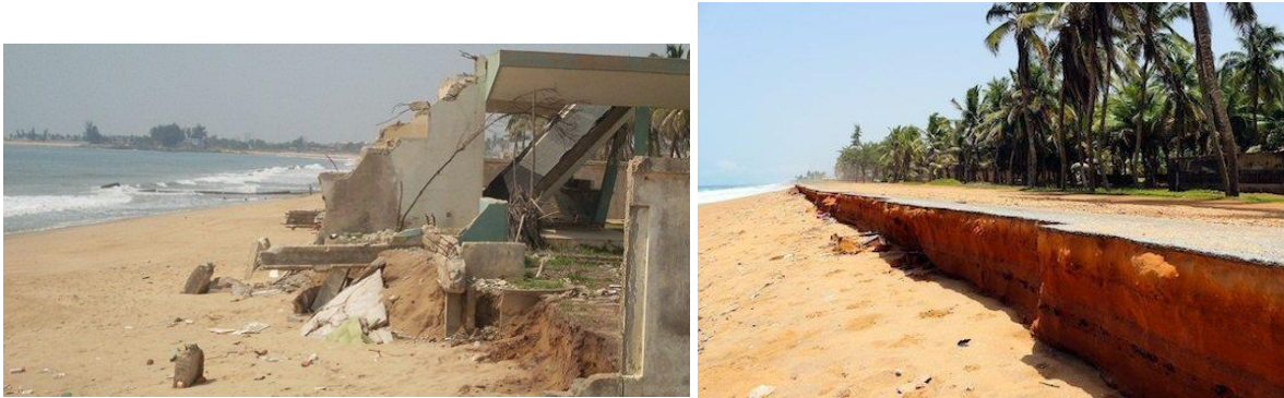
Manifestations of coastal erosion in Togo
